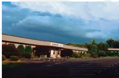
North Carolina Facility (USA)
