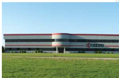
Ohio Facility (USA)
