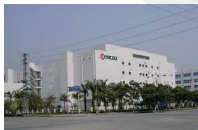
Silong Facility (CHINA)
