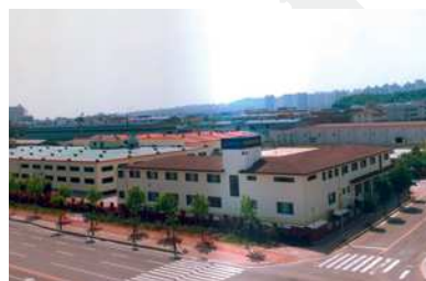
Incheon Facility (KOREA)
