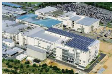
Yokaichi Facility (JAPAN)
