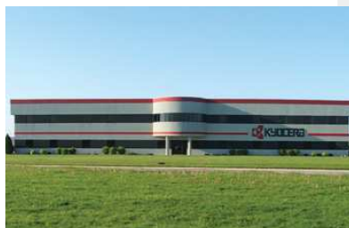
Ohio Facility (USA)
