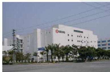
Silong Facility (CHINA)
