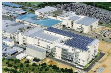
Yokaichi Facility (JAPAN)
