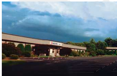
North Carolina Facility (USA)
