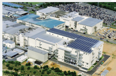
Yokaichi Facility (JAPAN)
