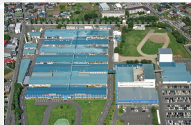
Okaya Facility (JAPAN)
