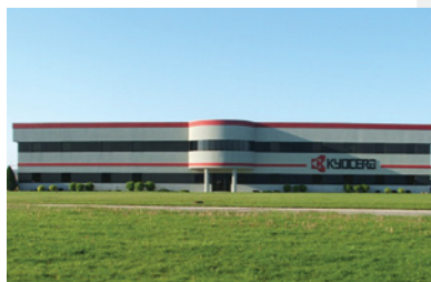
Ohio Facility (USA)
