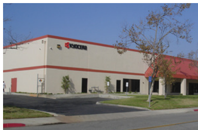
California Facility (USA)
