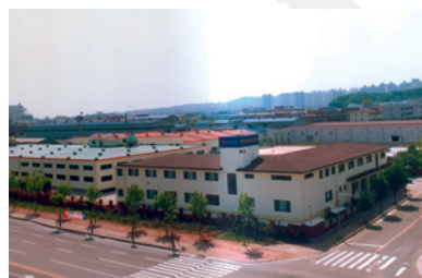
Incheon Facility (KOREA)
